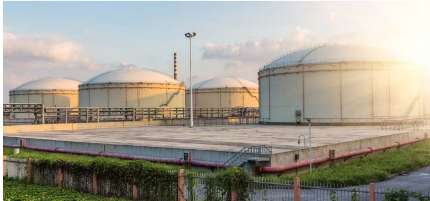
Biogas facilities help generate electricity and heat
