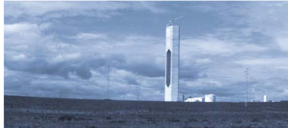
Method 1: Heliostat solar-thermal power plant
